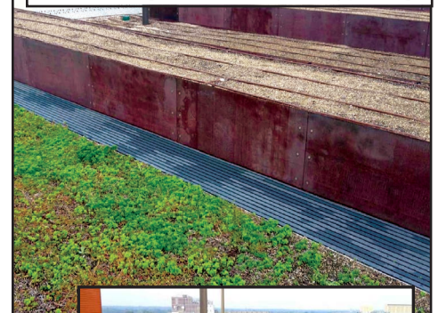
Fibergrate® gratings were used for drainage and walkways in front of the planter boxes on this rooftop green space. Molded grating was also used to make a storage area more aesthetically pleasing.
