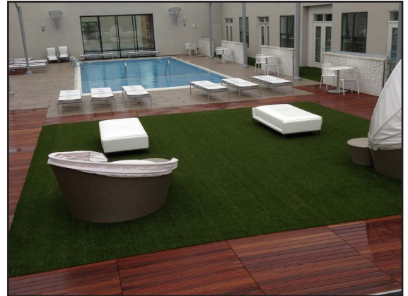
Fibergrate molded grating was used with Bison Pedestals to hold the grating, along with stone and wood pavers, used on the roof of this luxury apartment building. Artificial turf was placed over the grating resulting in low maintenance green space along walkways and in seating areas. The open mesh of the grating will allow for proper drainage and will not rust or rot.
