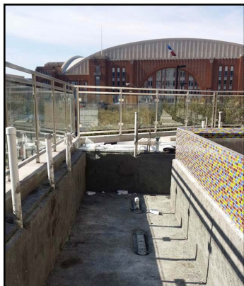
Fibergrate molded grating and quad head pedestal legs were used over this pool's drainage trench. It was then covered with a synthetic mesh, as an added filter for trash and debris, before being covered with river stones and walking pavers. This resulted in a secure walkway around the exterior of the pool while also allowing for proper drainage of overflowing water.
