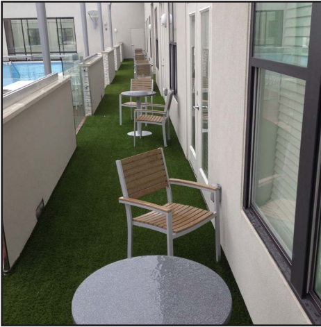
Fibergrate molded grating was used with Bison Pedestals to hold the grating, along with stone and wood pavers, used on the roof of this luxury apartment building. Artificial turf was placed over the grating resulting in low maintenance green space along walkways and in seating areas. The open mesh of the grating will allow for proper drainage and will not rust or rot.
