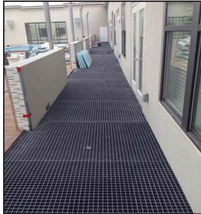
Fibergrate molded grating was used with Bison Pedestals to hold the grating, along with stone and wood pavers, used on the roof of this luxury apartment building. Artificial turf was placed over the grating resulting in low maintenance green space along walkways and in seating areas. The open mesh of the grating will allow for proper drainage and will not rust or rot.
