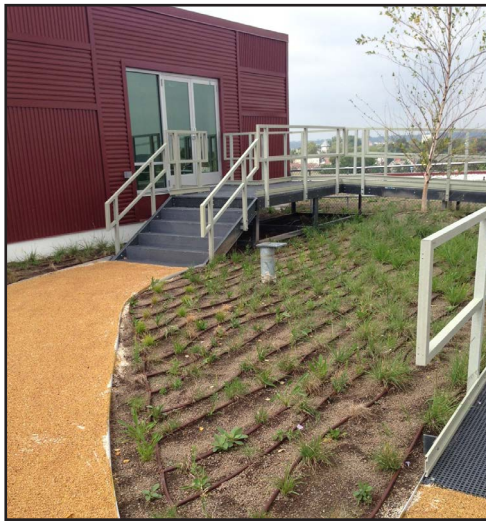
The final space includes Fibergrate's FRP rooftop walkway surrounded by live vegetation.
